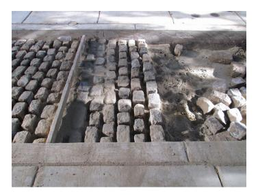
I'm glad I had a look. I'd never seen a reconstruction of a Belgian block street (above). It was a pretty elaborate thing. There was a concrete sub-pavement that joined seamlessly to the concrete curbs, forming a sort of bathtub without a drain. On the sub-pavement the workers laid a layer of sand; on this they placed the Belgian blocks, well spaced; and then they poured more sand into the seams between the pavers.
